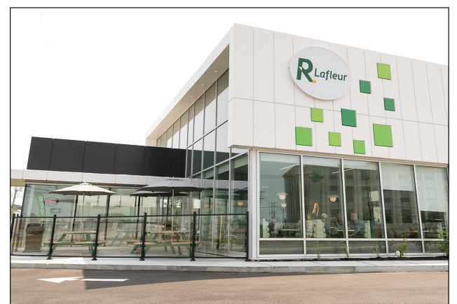
The revamped Lafleur Restaurant on Côte de Liesse
