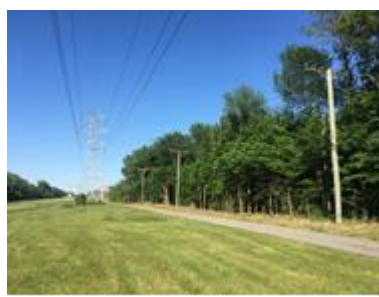
The same right-of-way after work
