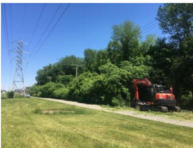
Transmission line right-of-way during work
